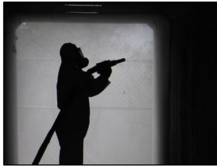
Sandblasting by Southern Paint
